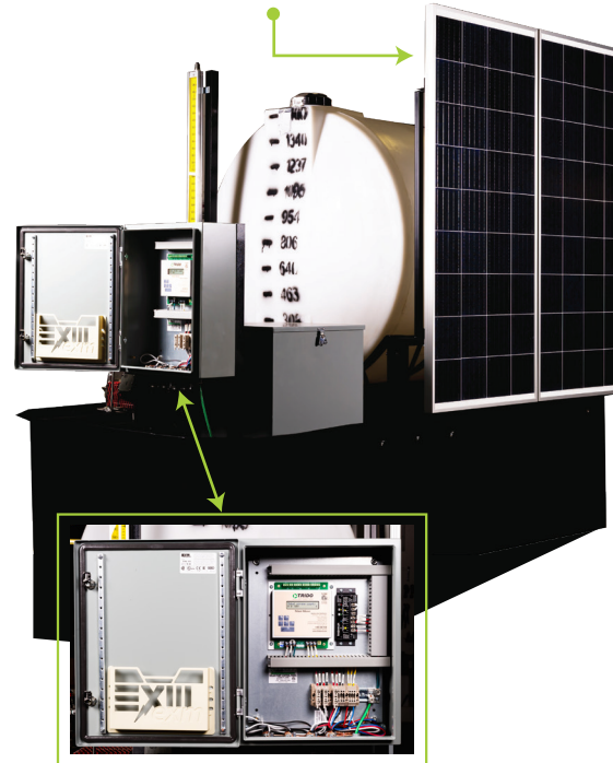
TRIDO MINI-MIZER CONTROLLER IN NEMA 4 ENCLOSURE
